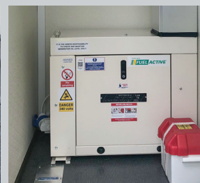
Warm room/ Generator area
